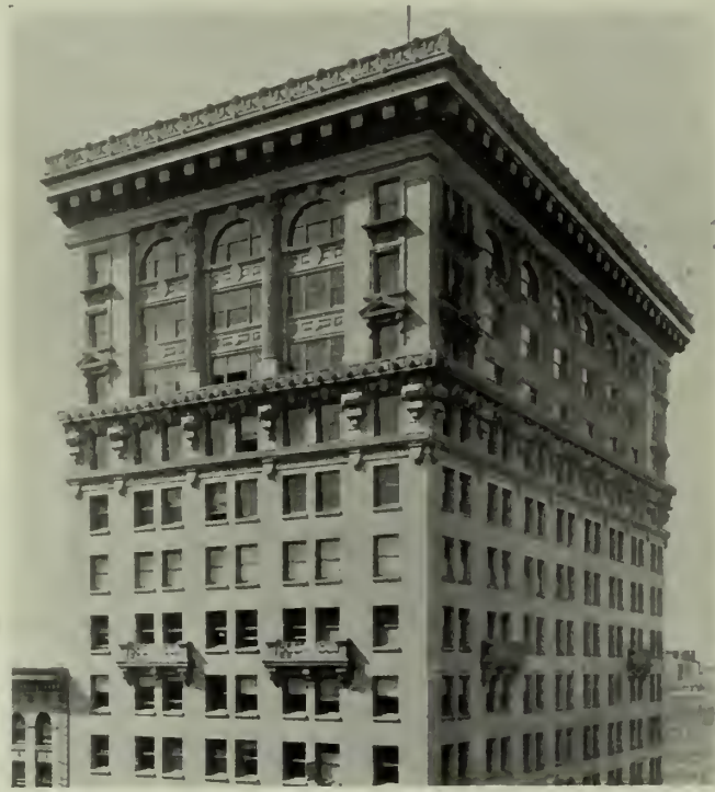
UPPER STORIES, MERCHANTS' EXCHANGE BUILDING, NEW YORK CITY.
